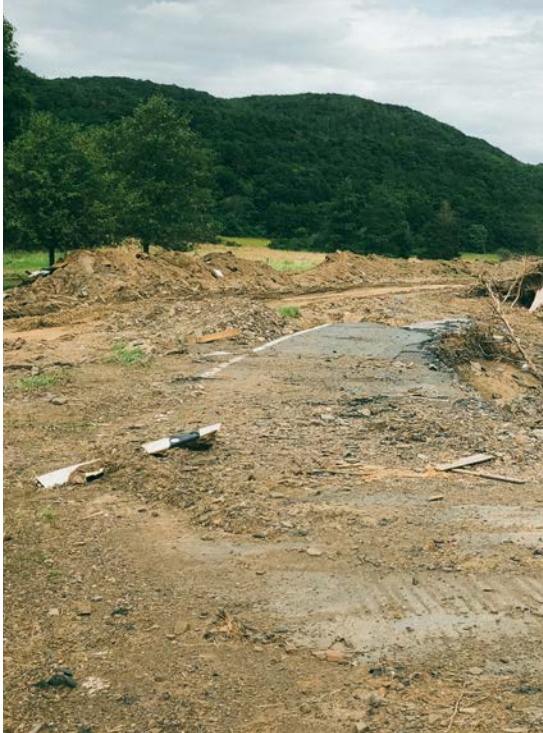
Surveying a section of road washed away by the Sahrbach.
