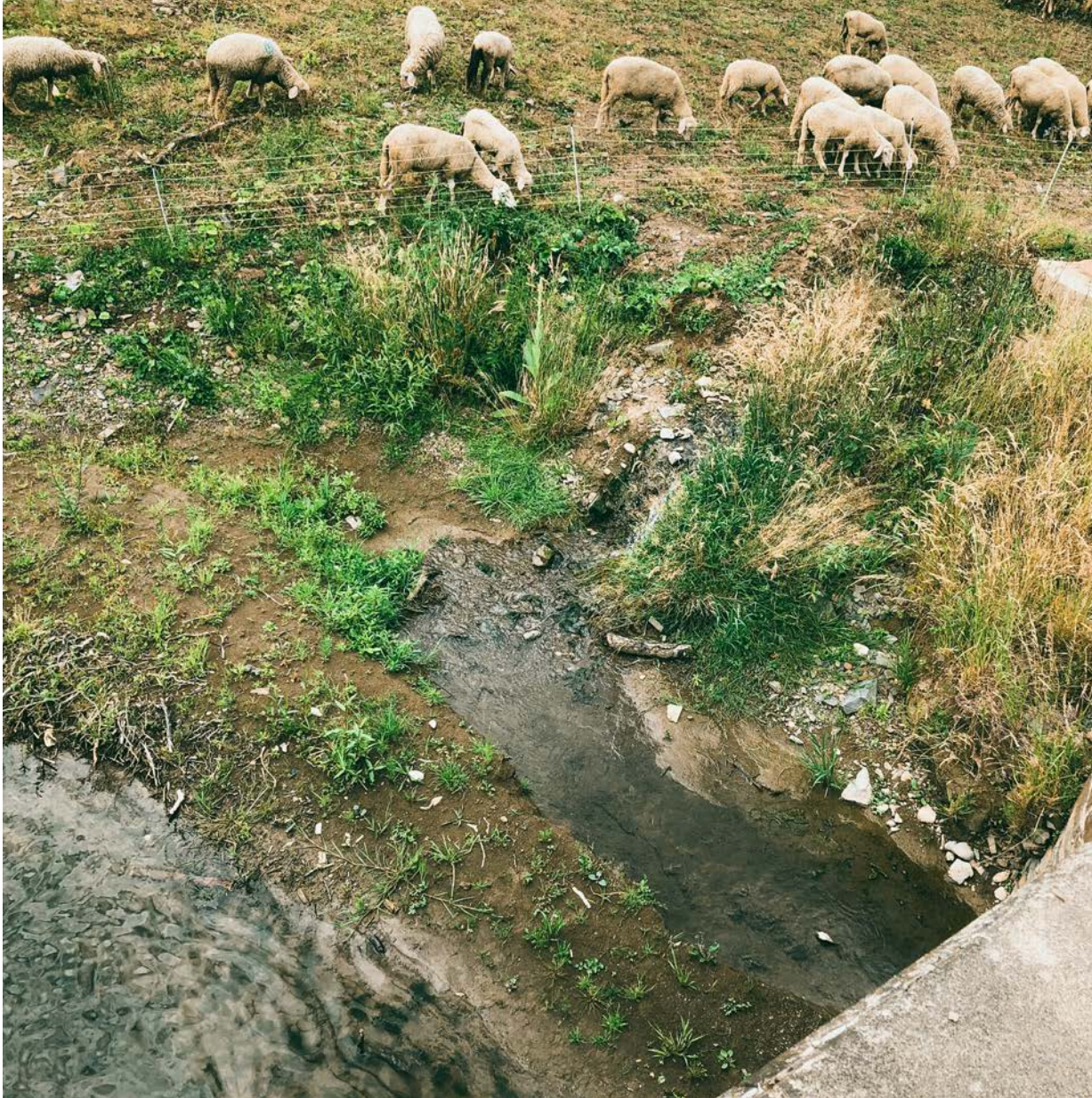
In 2022, raw sewage is still leaking into the Ahr.
