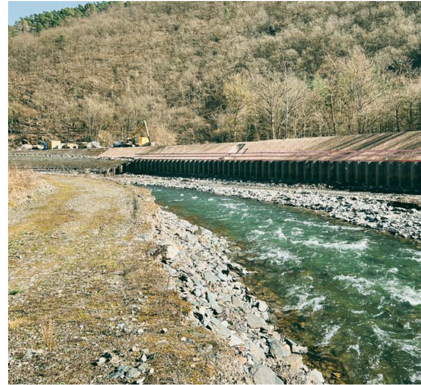
In early 2025, the noise of railway reconstruction echoes across the valley.
