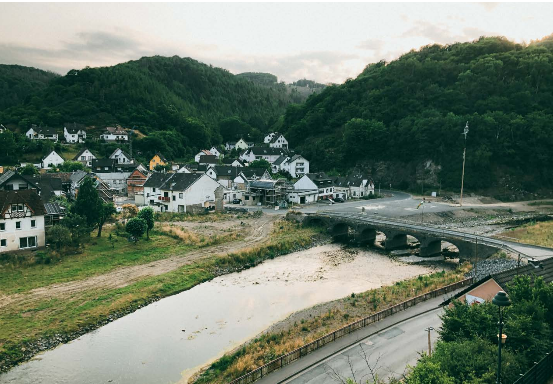
The damaged bridge connecting Brück and Ahrbrück in 2022.
